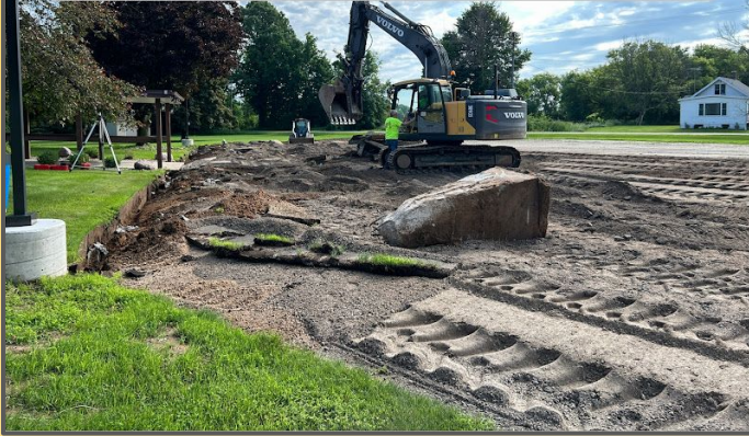
Mon, 6/30, 8:51am Curb and light pole base demo-ed
